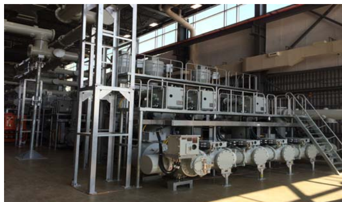
Photo: HICO 145kV Gas Insulated Switchgear
